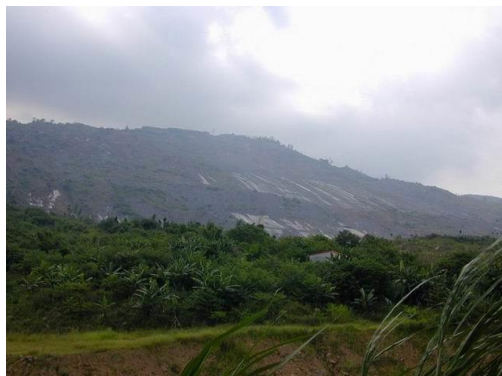
圖9 九份二山震災後之裸露坡面(2000/7/2) Figure 9 Earthquake-induced landslide site of the studied area on 2000/7/2
