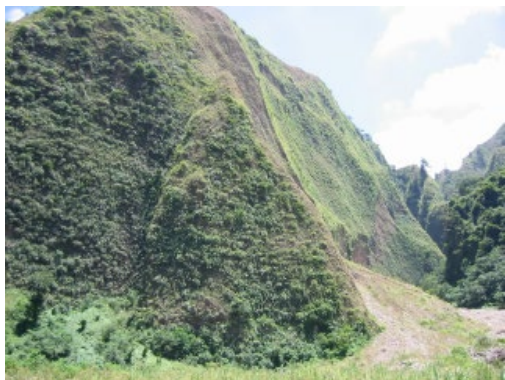
圖9 九九峰震災4年後崩塌地植生復育情形 Figure 9 Vegetation restoration condition of the landslide sites 4 years after the 921 earthquake
