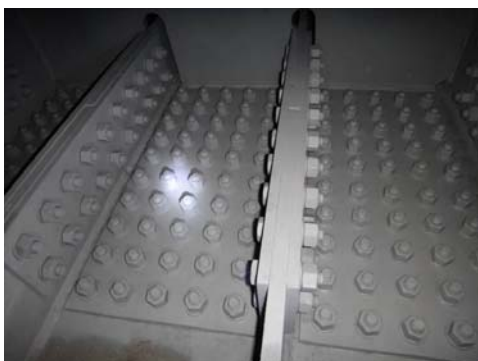
圖 3-12 高張力螺栓、油漆面檢測結果未發現異常 Fig. 3-12 High tensile bolts, paint surface has normal test results
