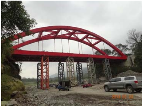
圖 3-17 支撐架安裝完成進行更換作業 Fig. 3-17 The replacement work for supporting frame installation has been complete
