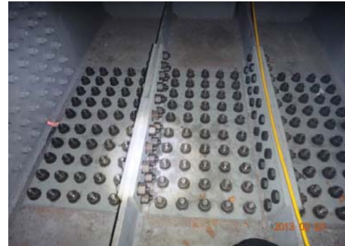
圖 3-19 接合鈑、高張力螺栓更換完成 Fig. 3-19 Replacement of bonding sheet and high tensile bolts were completed
