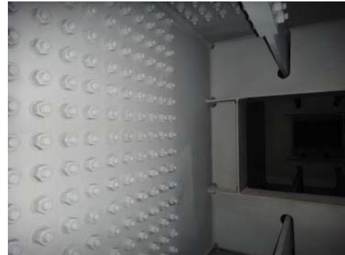
圖 3-13 高張力螺栓、油漆面檢測結果未發現異常 Fig. 3-13 High tensile bolts, paint surface has normal test results
