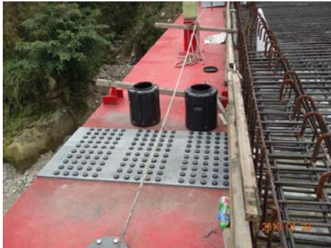
圖 3-16 箱樑上翼接合鈑、高張力螺栓更換 Fig. 3-16 Both the Box on the wing joining sheet and high tensile bolts were replaced
