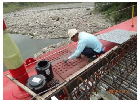
圖 3-15 箱樑上翼接合鉸高張力螺栓拆除 Fig. 3-15 Box on the wing joining sheet metal high tensile bolts were removed
