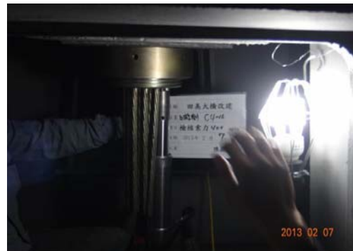
圖 3-20 鋼索預力重新調整 Fig. 3-20 Re-adjust the prestressing wire rope
