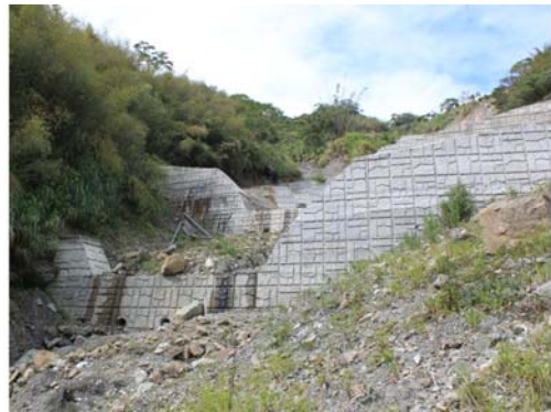
圖 13 崩塌地下游側既有防砂壩 Figure 13 A check dam at the downstream of the Laitou Creek
