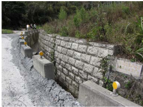
圖 12 崩塌地內之既有排水系統 Figure 12 The drainage system in the landslide
