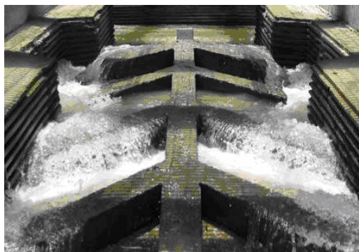
Figure 4. The fish passage for aquatic life at the Long-En-Yan diversion (courtesy Water Resources Agency)
