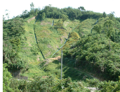
圖 8c. 崩場地處理現址-施工後(三灣鄉) Figure 8c. After construction.
