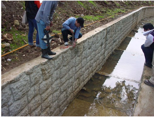
圖 14. 開口式及封底式交錯排列之溝水溝 Figure 14. Checking the newly constructed drainage structure.
