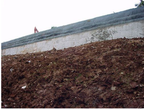
圖 7. 邊坡崩塌後現地施工現場 Figure 7. Repair work for slope failed.
