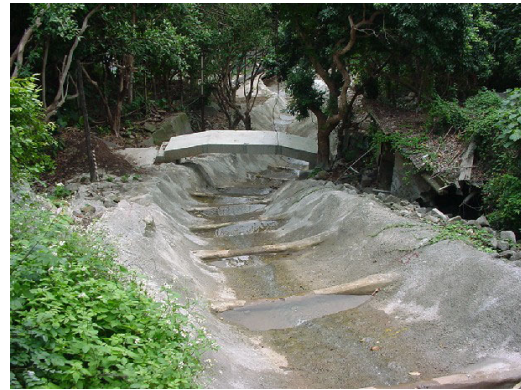
圖 15. 噴漿排水溝 Figure 15. Concrete drainage channel.
